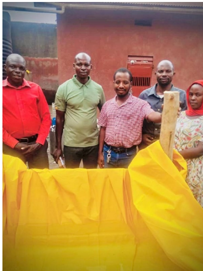
A timber-supported, tarpaulin-lined pool prepared at Kagadi Prison.
